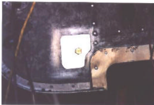
Initial Fit Up of Flush Patch using Bolt for Centering - Left Hand Engine Firewall Shown - Right Hand Firewall Similar.
